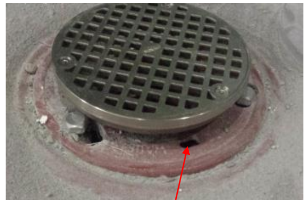
Weep hole in drain typically 3 or 4 in the top of the drain flange.
