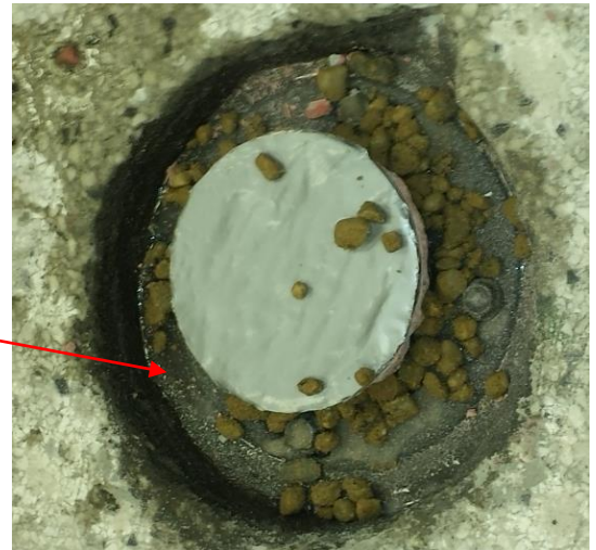
Pea gravel surrounding weep holes
