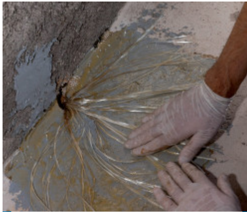
The splayed end of a piece of MapeWrap Fiocco cord
