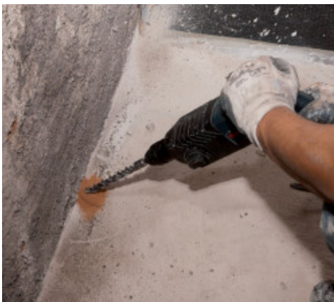
Drilling the hole
