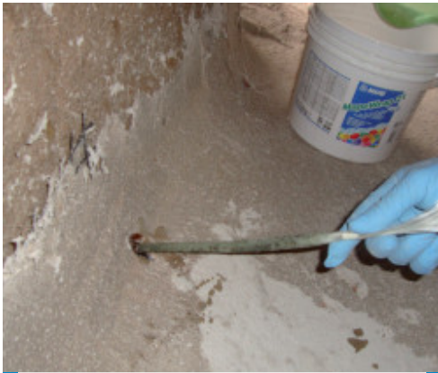
Inserting MapeWrap Fiocco cord in the hole
