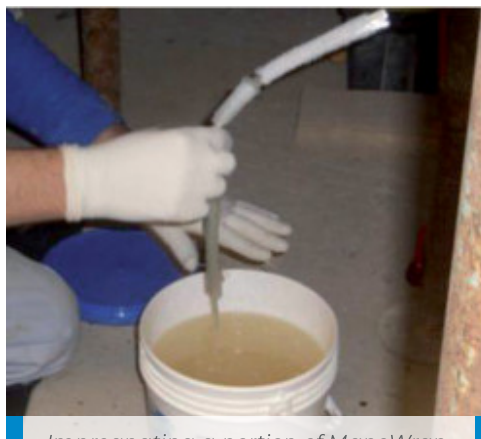
Impregnating a portion of MapeWrap Fiocco cord
