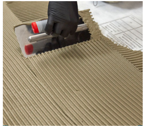
Used over Mapeguard 2
