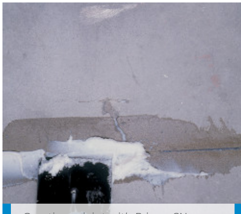
Grouting a joint with Primer SN admixed with Additix PE
