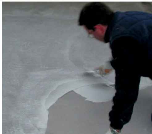
Primer SN thickened with Additix PE
