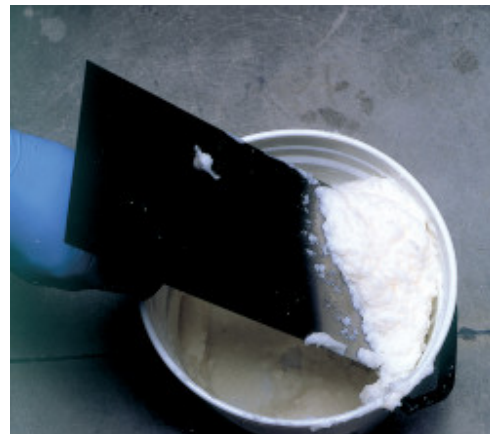
Mixing Additix PE in Primer SN
